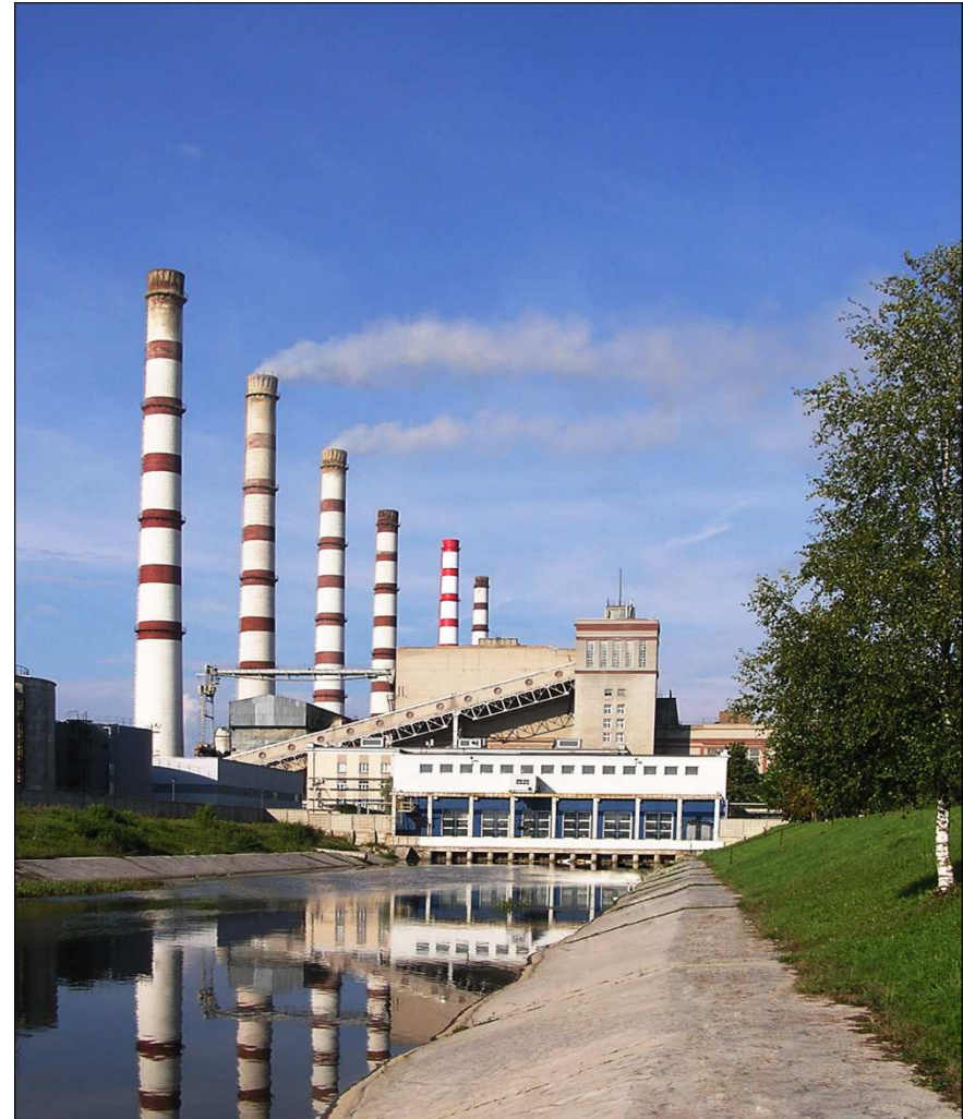
BALTI POWER PLANT
